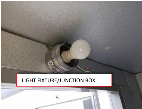
REMOVE SCREWS TO ACCESS JUNCTION BOX
