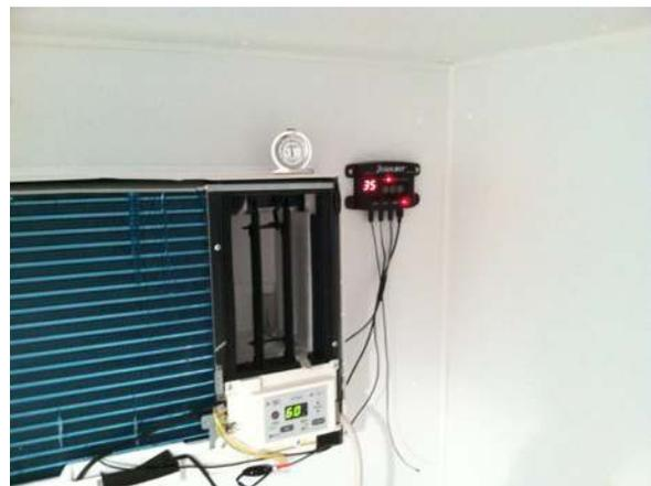
We set the Coolbot for 35 degrees and turned on the ac with the fan setting on high, as instructed in the Coolbot manual.
