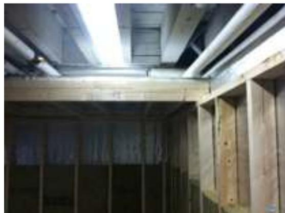
If you notice in the above photos, we laid the 2" insulation all the way down the outside of the floor, then built the wall frame on the floor itself, so we would not have any leaking of cold air. We also caulked heavily around these areas to make it airtight.
