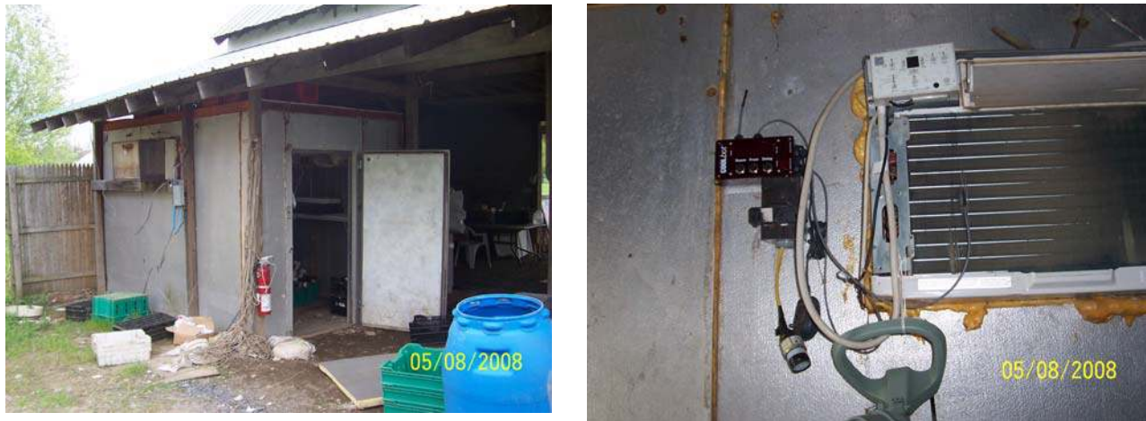
Figure 3. Photos of Metal-skinned Cooler Built Inside Pole Barn
